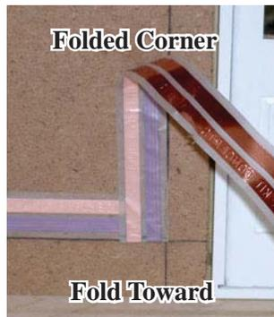
The simple sponce run<sup>1</sup> is the traditional style of connecting tapewire runs, eyeleted on one end. For more robust wiring, hook each run into the wiring on both ends<sup>2</sup> (copper-to-copper and blue-to-blue!)
