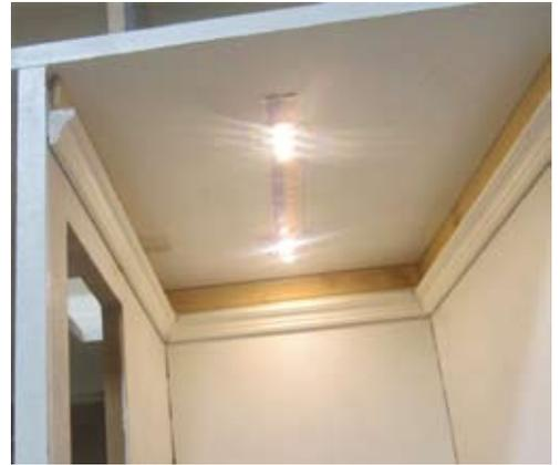
Test - if it doesn't light, you may have to switch the wires at the transformer (to make the copper the "+" leg of the wire).
