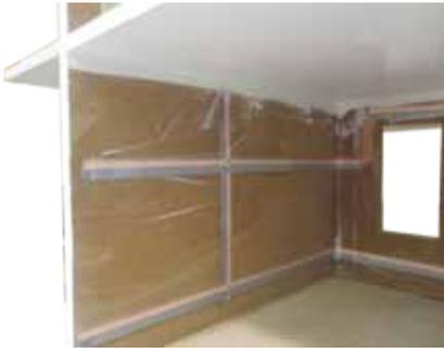
A thoroughly wired house (the Sconce Run will not be used). **Note the blue lead is toward the back on the vertical tapewire.**
